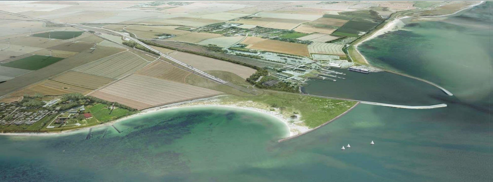
Future tunnel area Puttgarden
