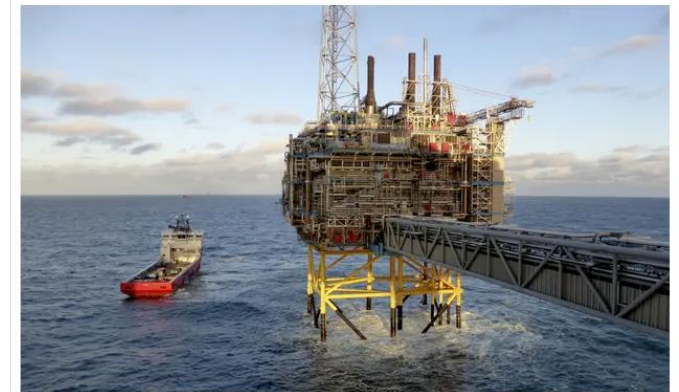
▲ Statoil gas processing and CO2 removal offshore platform near Stavanger, Norway. Photograph: Reuters Staff/Reuters
