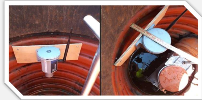
Level measurement inside a well
