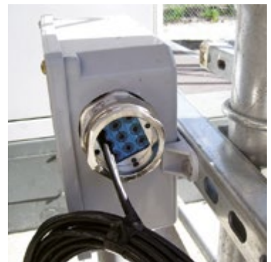
Telecom cabinet: The Roxtec RG M63 cable glands are weather, water, pest and dust tight.
