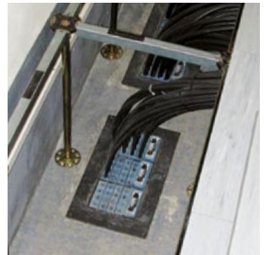
Communication centers: The Roxtec GHM solution seals fiber optics and cables in floors and outer walls.
