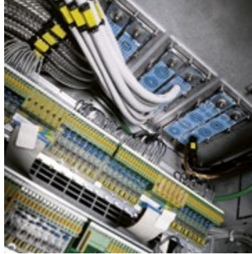
I/C cabinets: Neat and area efficient cable entry seals suitable for safety and non-safety applications.
